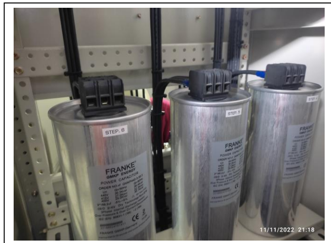
Picture 9: Ground & Capacitors Banks Preventive maintenance.
