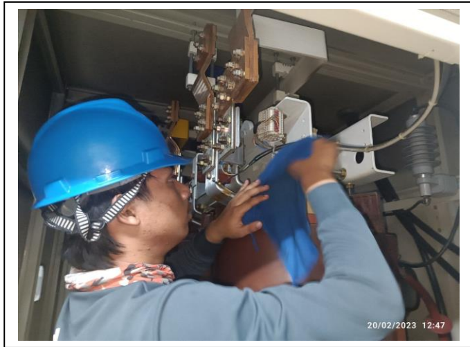
Picture 2: Cast resin Dry type Transformer and preventive maintenance.
