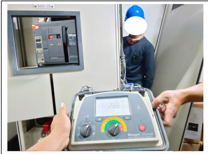
Picture 6: Air circuit Breakers and preventive maintenance.
