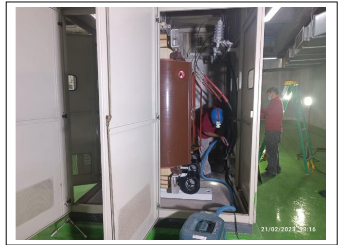
Picture 3: Cast resin Transformer and preventive maintenance.
