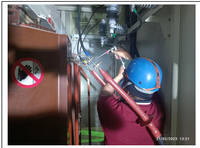
Picture 3: Cast resin Transformer and preventive maintenance.
