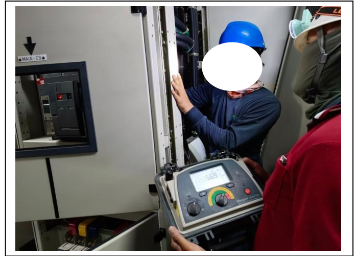
Picture 6: Air circuit Breakers and preventive maintenance.
