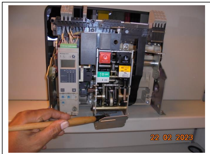
Picture 7: Air circuit Breakers and preventive maintenance.
