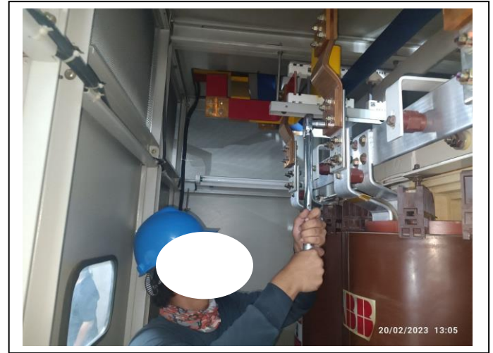
Picture 2: Cast resin Dry type Transformer and preventive maintenance.
