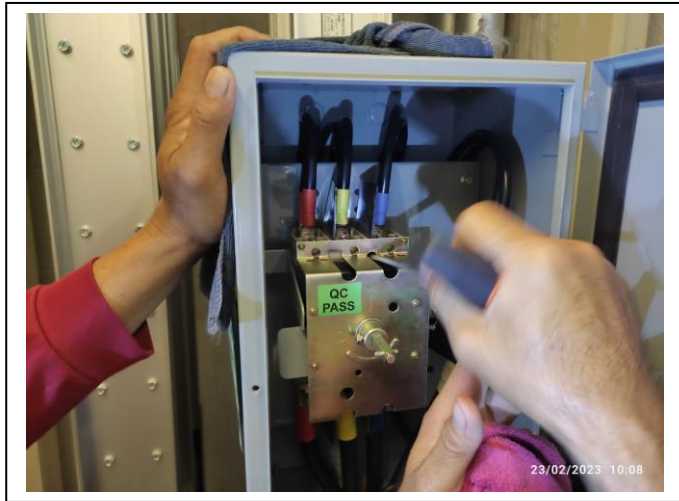
Picture 10: Distribution Board., Busduct Plug in & Preventive maintenance
