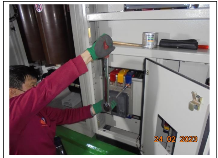
Picture 5: Main distribution board and preventive maintenance.
