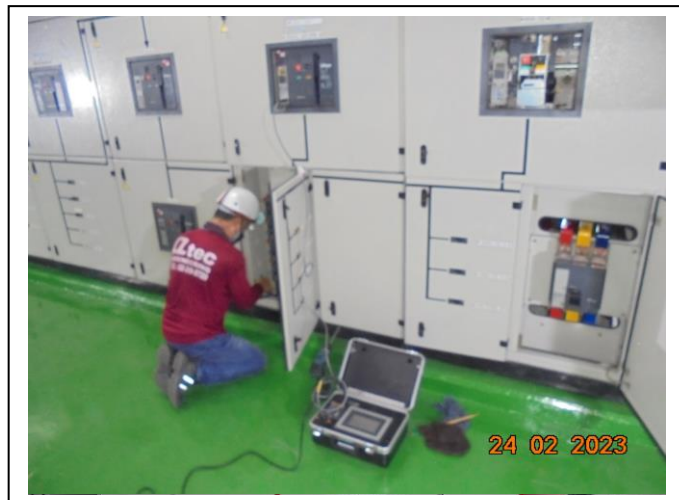
Picture 7: Air circuit Breakers and preventive maintenance.
