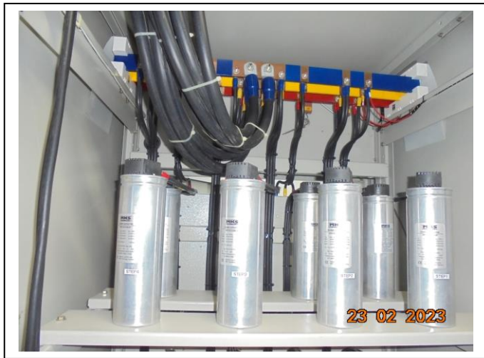
Picture 12: Capacitors Banks Preventive maintenance.
